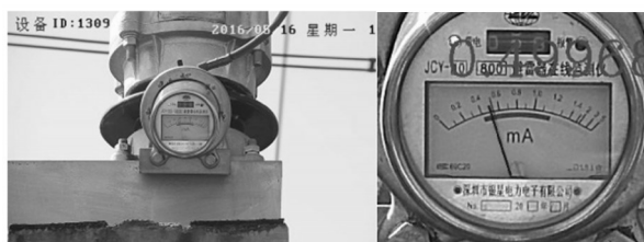
图21 避雷器泄漏电流表 Fig. 21 Leakage amperemeter of lightning arrester
