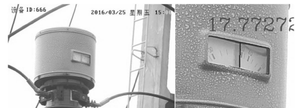
图23 油位表识别 Fig. 23 Oil level recognition
